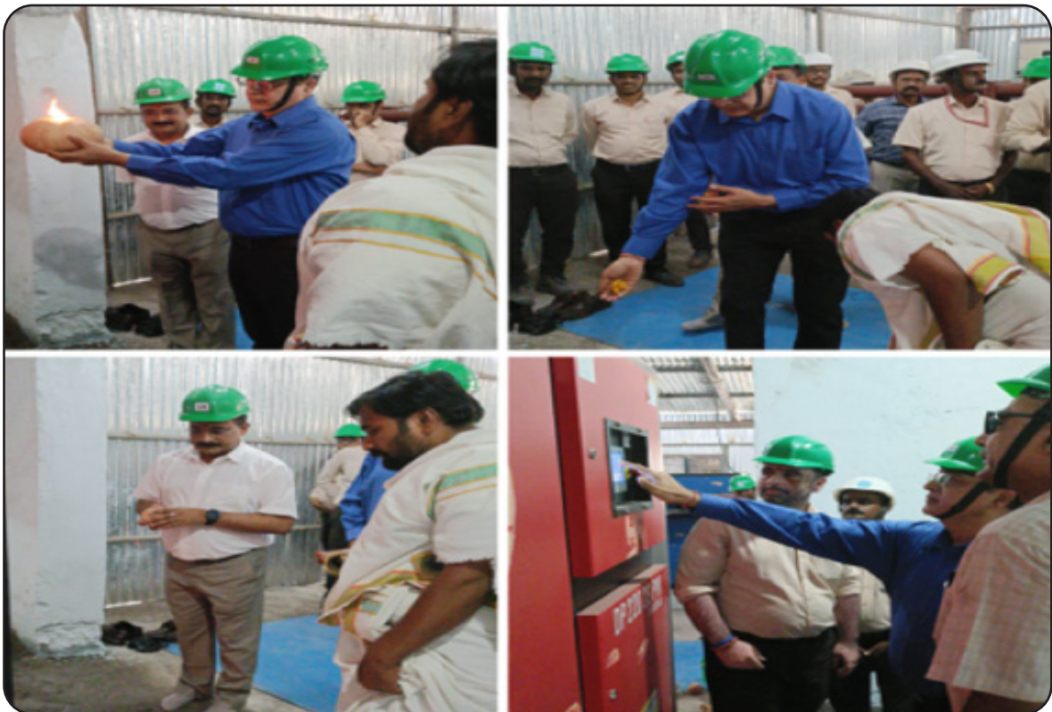
Inauguration of energy efficient Compressor under Demonstration of Energy Efficiency Project (DEEP) - Energy Efficiency Services Limited (EESL) at CCI Tander Factory By Hon'ble CMD,CCI
