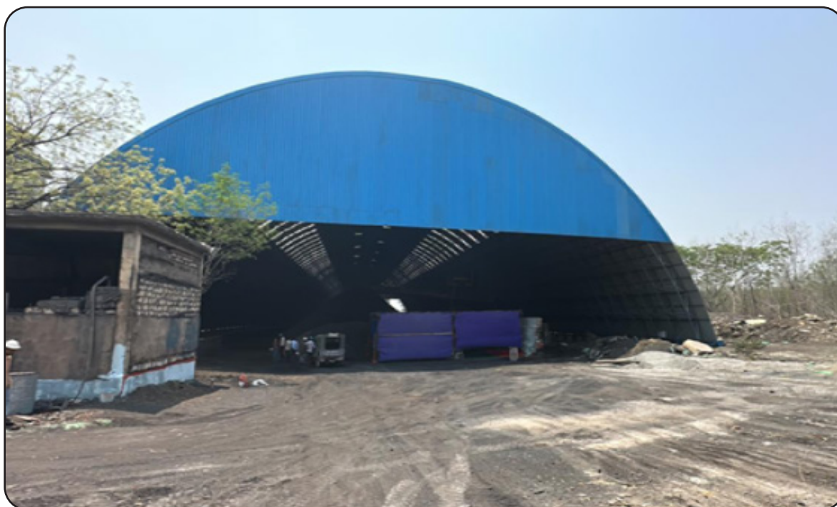
Coal Shed at Tandur (Reduction in Coal Consumption/Improve Plant Operation)
