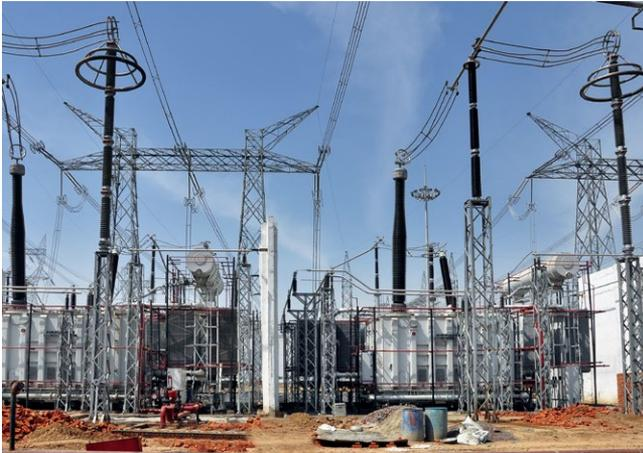
500 MVA 765/400/33 kV auto transformer at 765 kV Greater Noida substation
