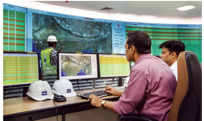
Central control room at Agra converter station of the world's largest ± 800 kV, 6000 MW UHVDC multiterminal North-East Agra transmission link, being executed by BHEL on turnkey basis
