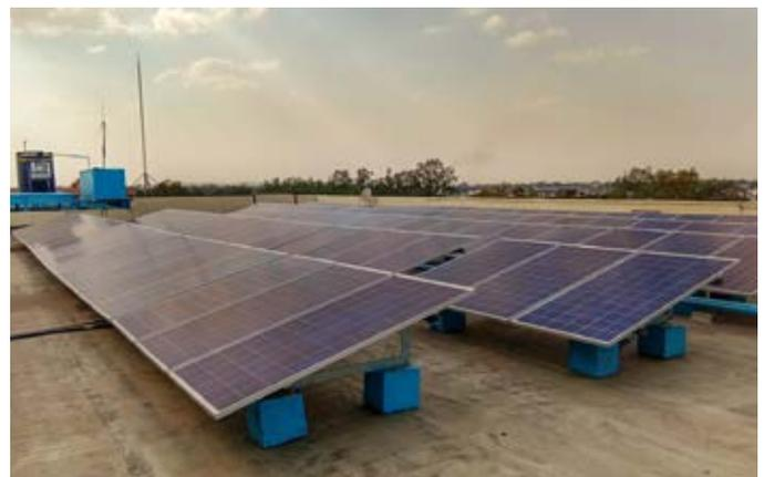
*295 kW<sub>p</sub> in-house developed Solar Rooftop SPV panel at BHEL Bhopal*
