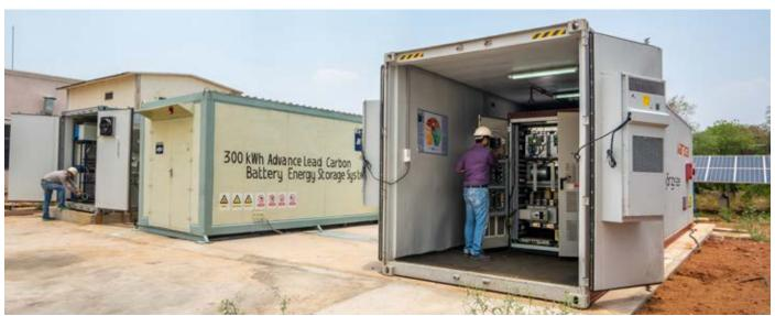
1MW Battery Energy Storage System (BESS) for in-house usage, developed & commissioned at Corporate R&D, Hyderabad
