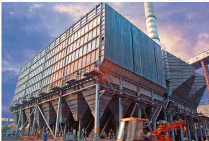
Addressing environmental concerns, BHEL has been manufacturing Electrostatic Precipitators for decades and is also now manufacturing FGD systems
