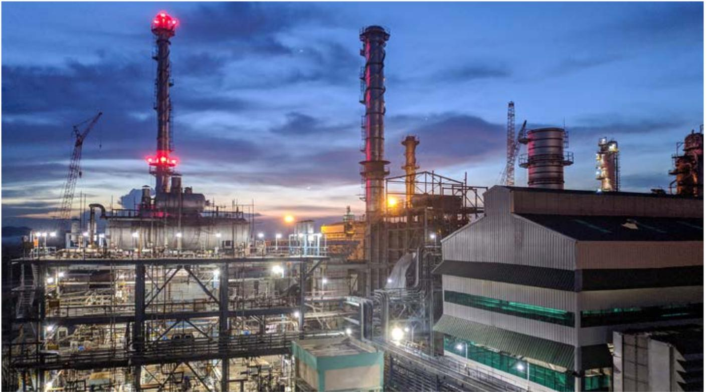
*RFCL Ramagundam CPP with 32.5 MW rating Gas Turbine along with Utility Boiler and Heat Recovery Steam Generator - under commissioning by BHEL in Telangana*
