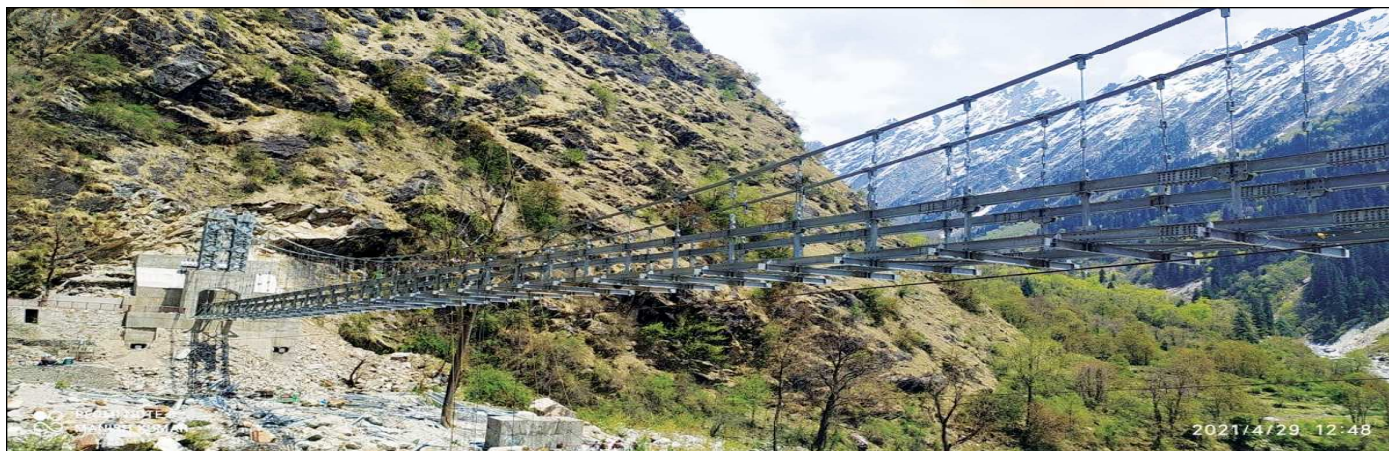
135-meter span Suspension Pedestrian Steel Bridge on Govindghat to Ghangharia Road at KM 10 in Chamoli District for PWD, Uttarakhand [B&R Project]
