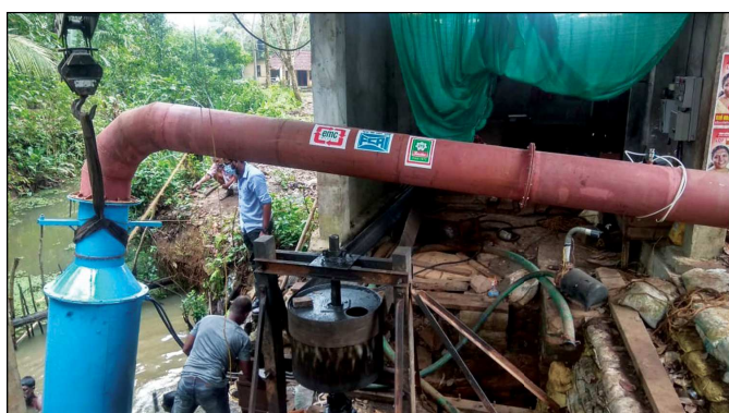
One of the axial flow submersible pumps in operation
